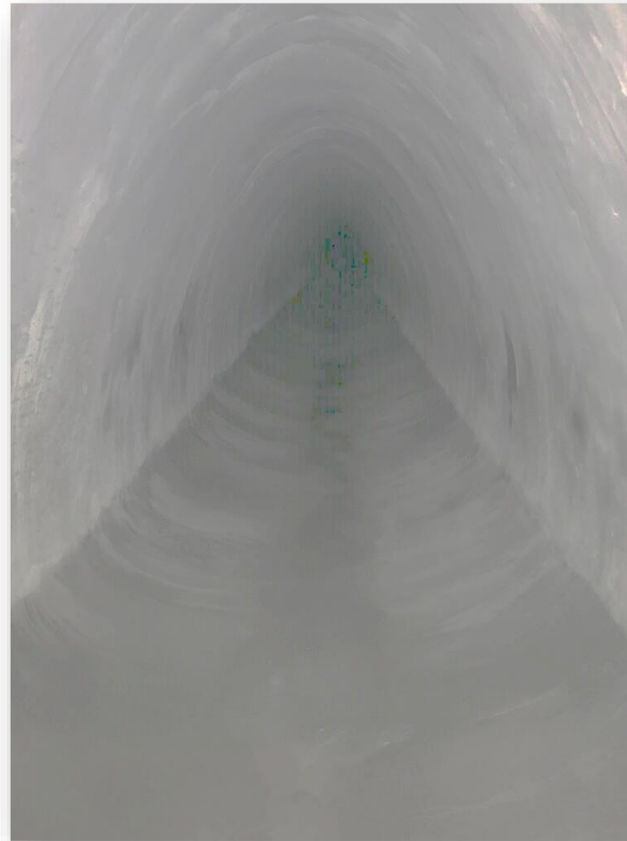
Pipe Structural Lining Completed
